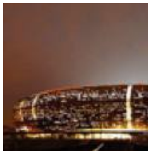
Soccer City Stadium Johannesburg (Afrique du sud) 2009
